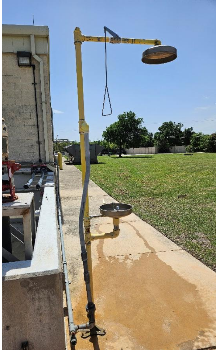
Figure 3-9: Emergency Eyewash Station
