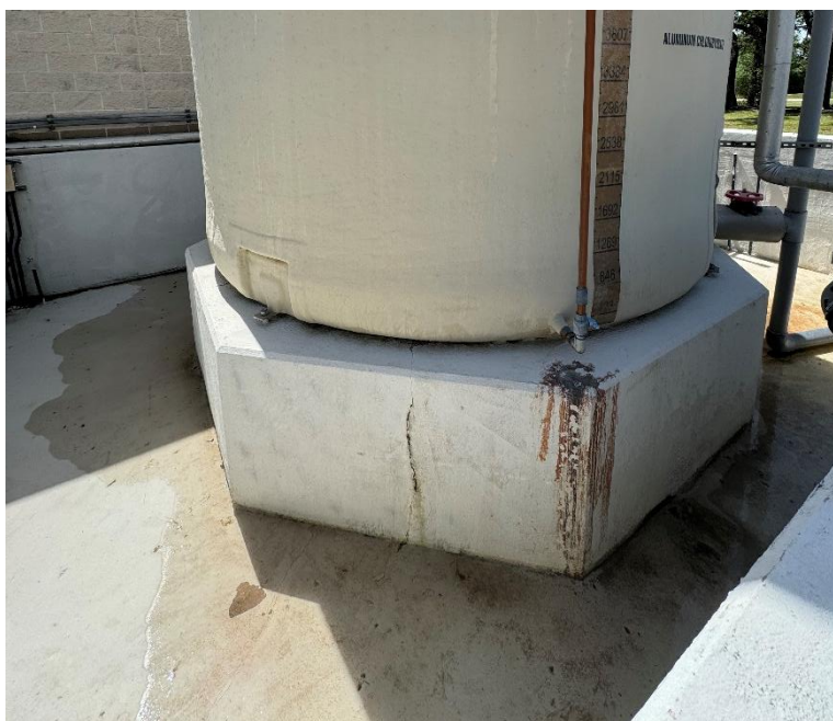
Figure 3-8: Standing Water in Outdoor Chemical Storage Area
