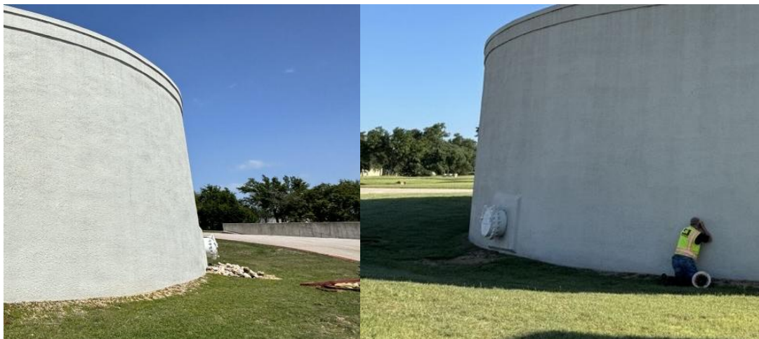
Figure 3-20: Clearwell Existing Drainage Infrastructure (Left: Clearwell #1, Right: Clearwell #2)
