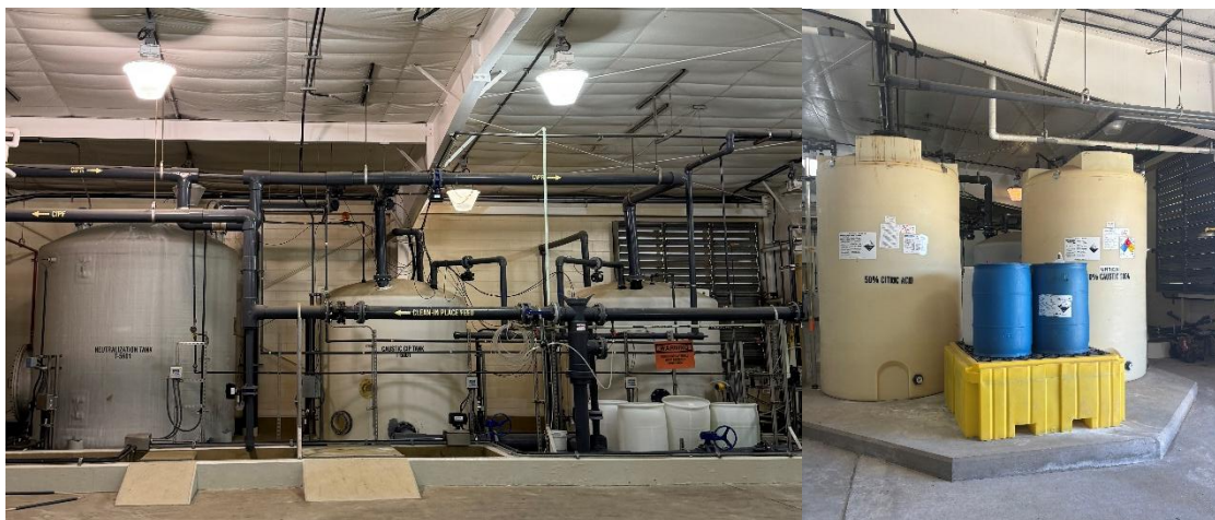
Figure 3-18: Clean-in-Place System
