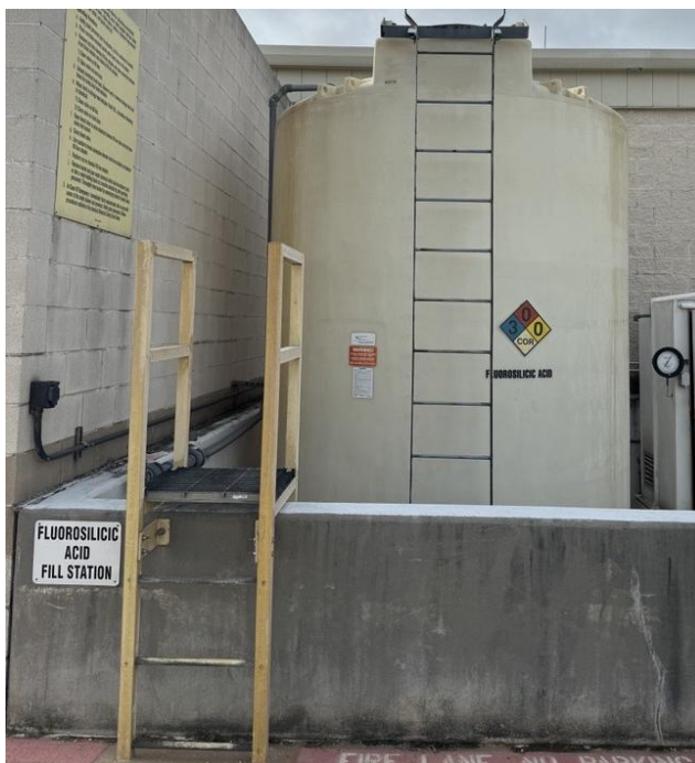
Figure 3-7: Fluorosilicic Acid Tank
