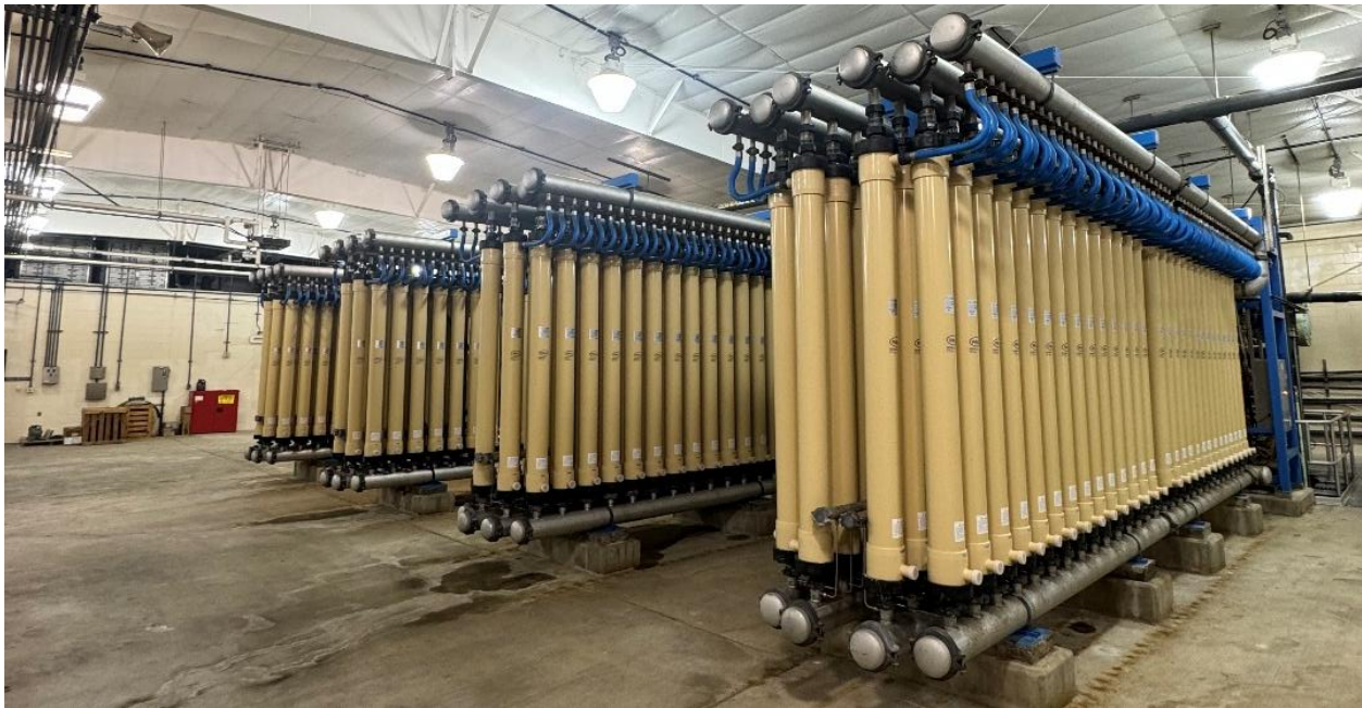
Figure 3-11: Pall Membrane Racks
