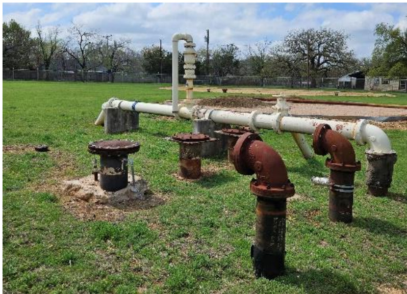
Figure 4-4: Unused Well 5 Piping to be Demolished
