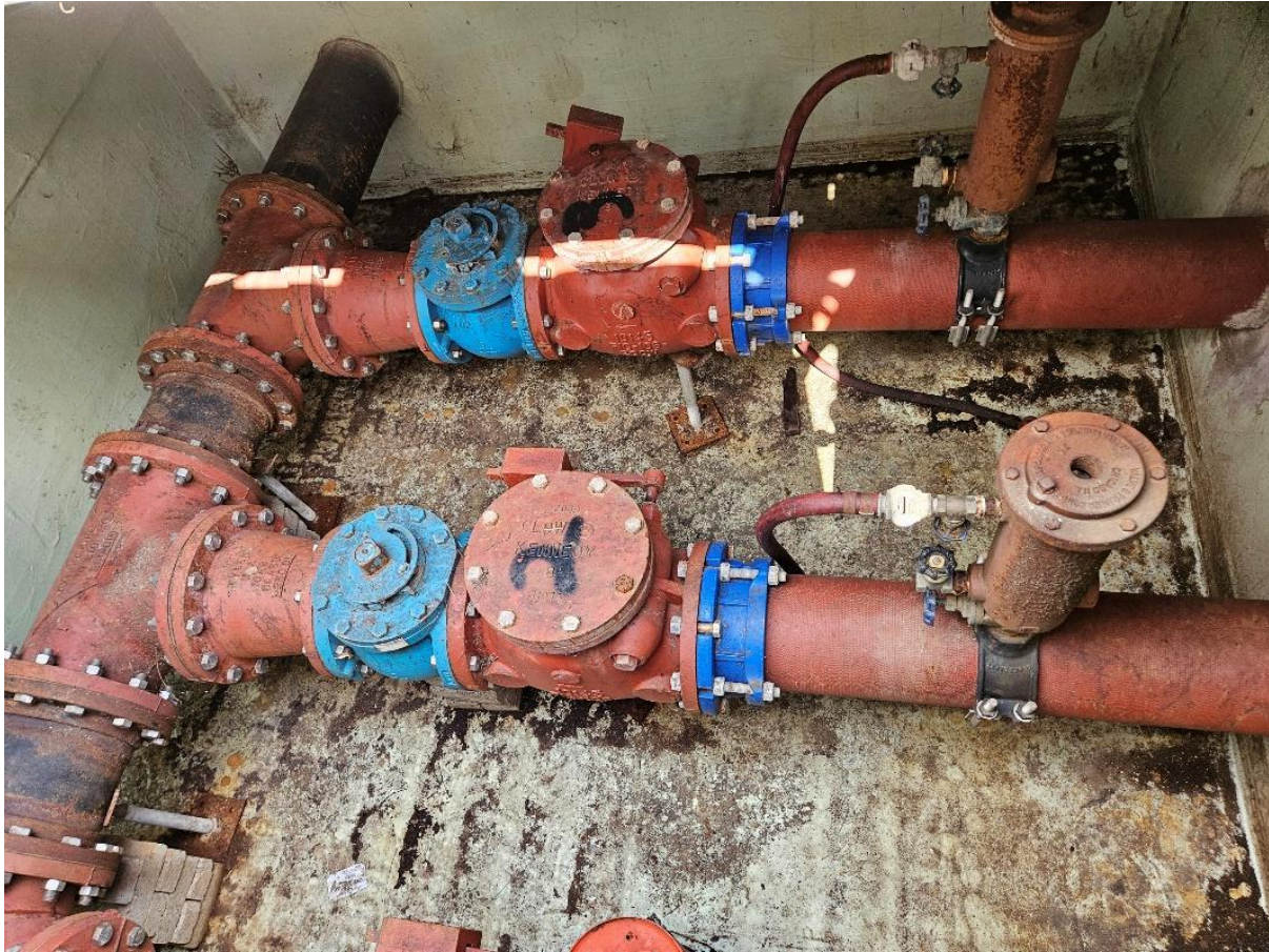
Figure 8-8: Highland Horizon I LS Pipe Stanchions
