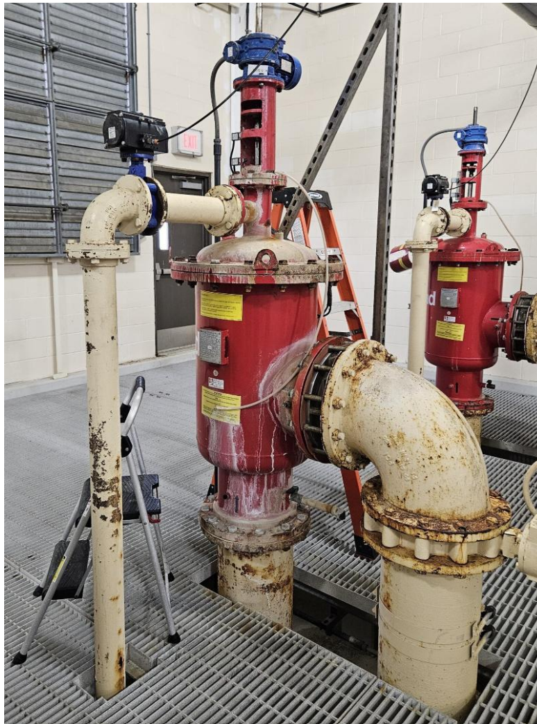
Figure 3-10: Amiad Strainers
