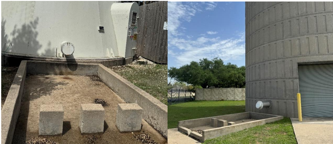
Figure 4-8: Elevated Storage Tank Overflow Systems (Left: North, Right: Neenah)
