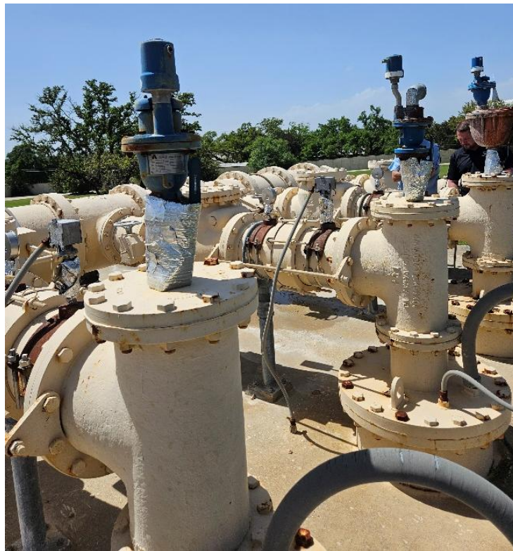
Figure 3-17: Membrane Feed Pumps
