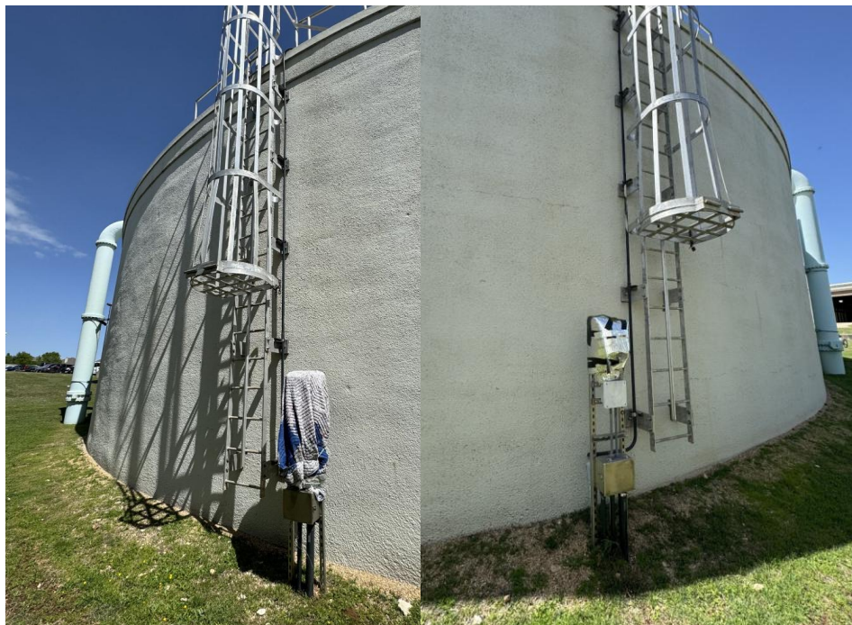
Figure 3-21: Clearwell Meters (Left: Clearwell #1, Right: Clearwell #2)
