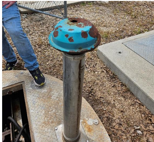
Figure 8-10: Highland Horizon II Corroded Vent
