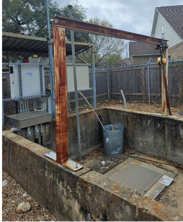
Figure 8-5: Liberty Walk Lift Station Jib Crane
