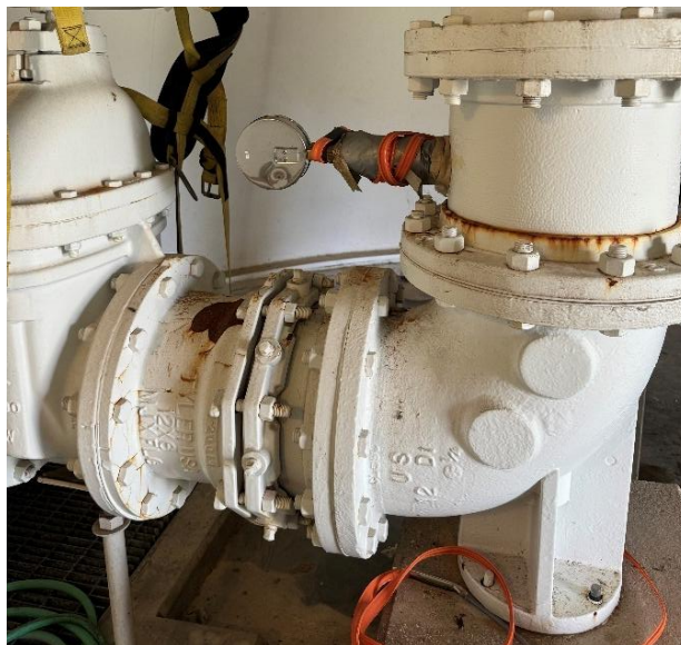
Figure 4-9: North Elevated Storage Tank Pipe Corrosion
